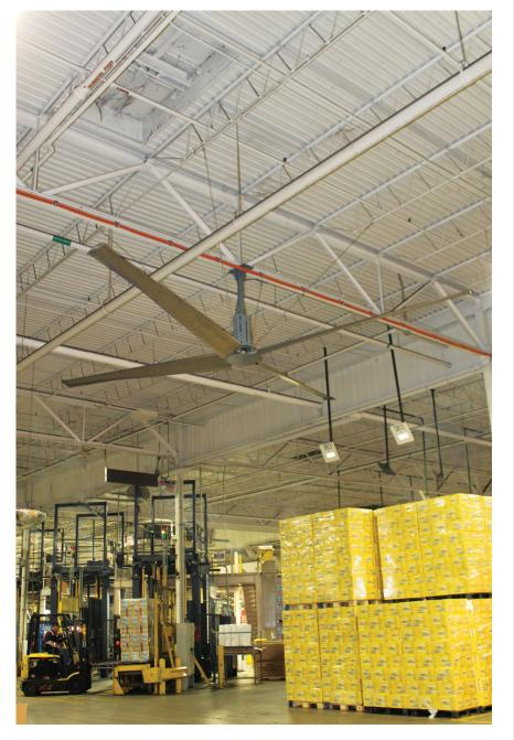
performance of different designs will vary in the uniformity of air movement directly below the fan, as well as the height and reach of air movement outward from the fan's diameter.
